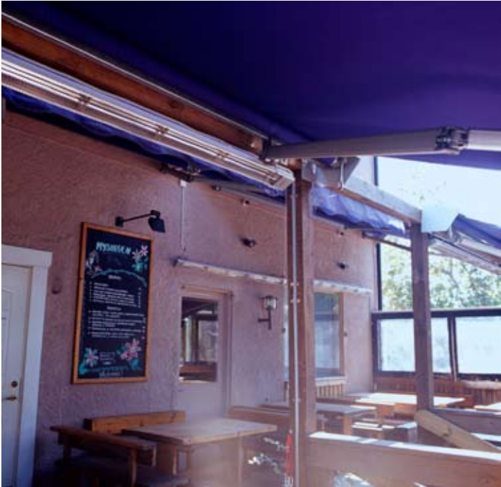
CIR is an ideal solution for giving comfort to customers at outdoor restaurants. The heaters can be mounted on the restaurant’s wall or in line directly above the tables in large terraces.
